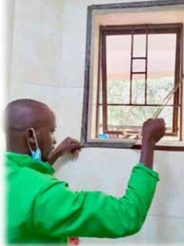
Mosquito netting attached to windows
