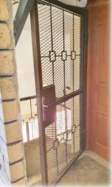
Meshed and grilled door to keep out the monkeys
