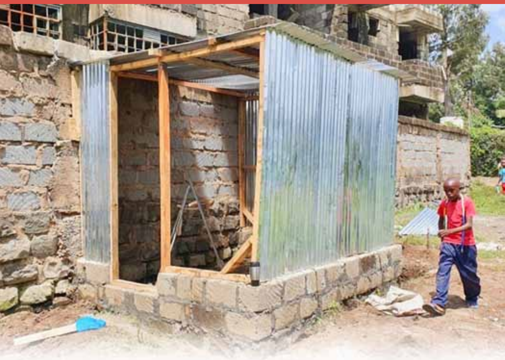
A small enclosure for the pump controller for the Rongai water project
