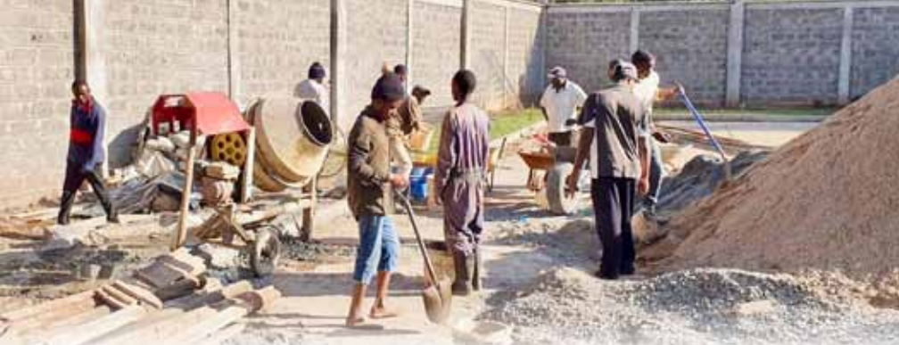
Concrete is poured for the base of a storehouse at the Karen residence
