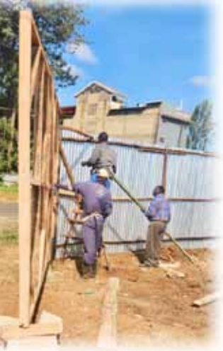
Erecting fencing around the Gachanka construction site
