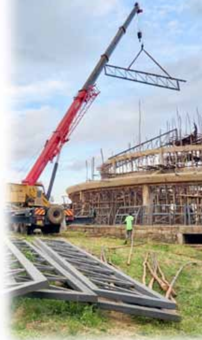
Lifting the roof into place for the Gachanka church
