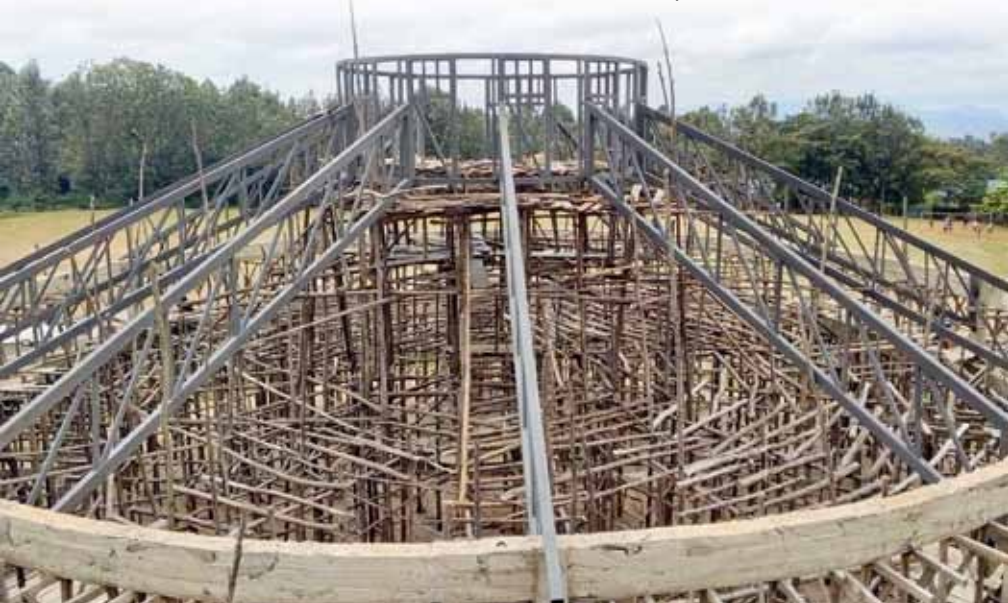
Gachanka church roof structure in place
