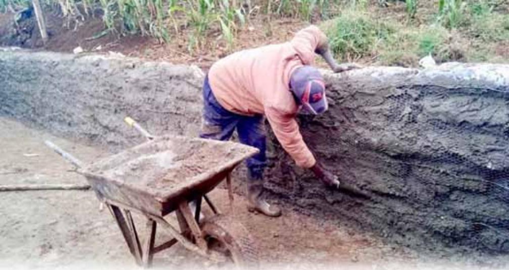
Plastering the retaining wall at Kiirua farm
