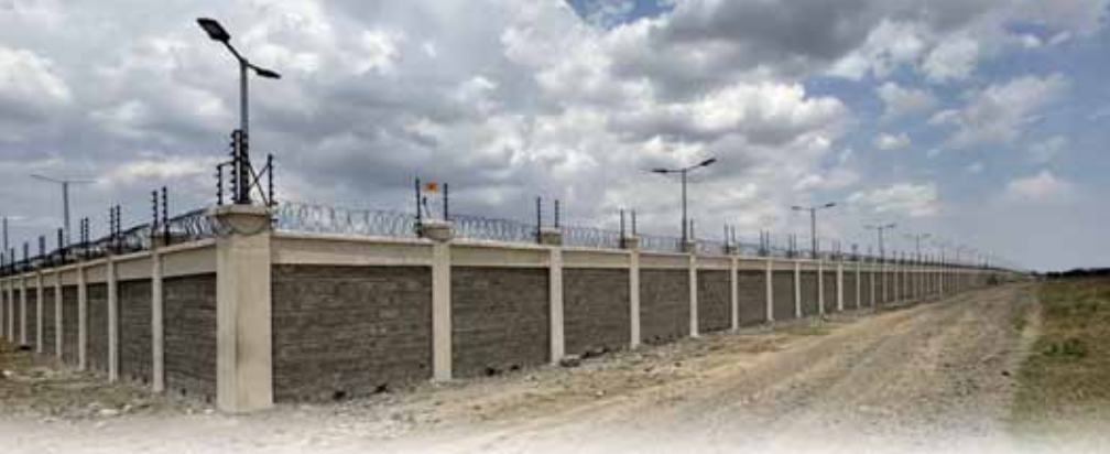
Perimeter wall at the university
