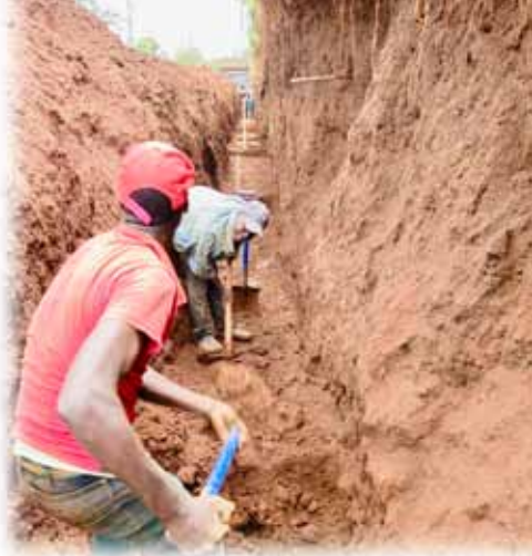
Irinda Wall foundation trenches
