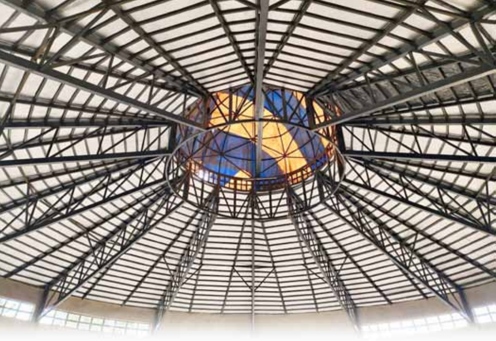
Gachanka Church in progress
