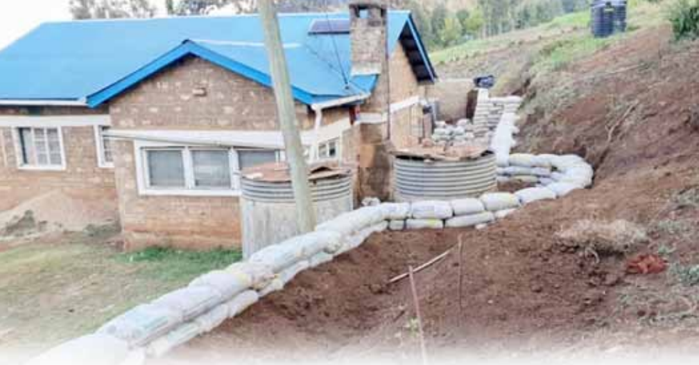
Retaining wall behind the house at Kiirua farm
