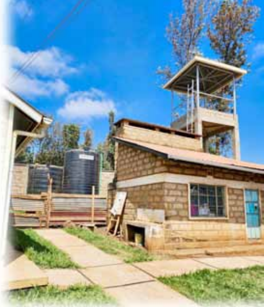
Completed water tower in Méru Parish
