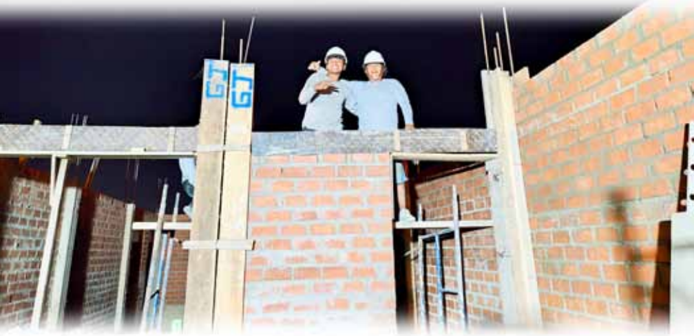
Home under construction in Peru
