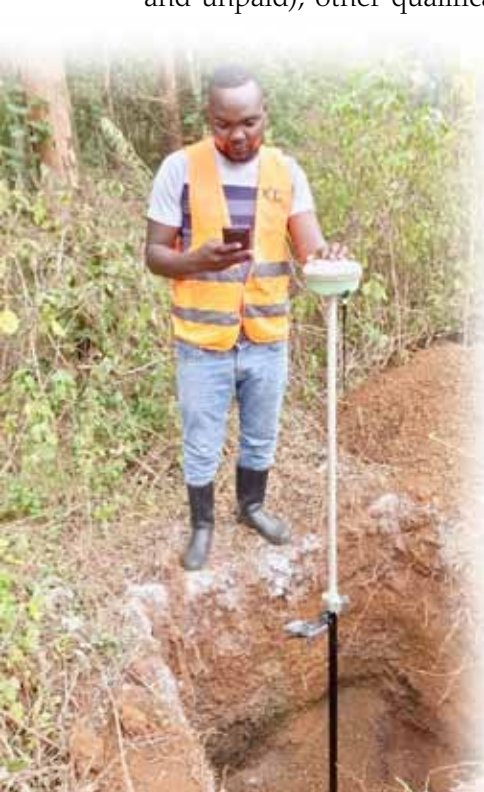
Survey work for boundary marking columns at Kiirua farm
